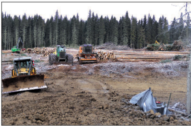
Construction at the site, on Nov. 20.
