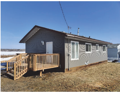
After photo of a house in Wabasca.
