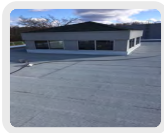
Calling Lake Roof Roofing Two years in a row
